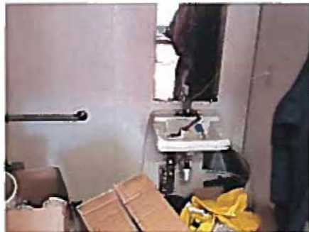
Existing Non-Functional Restroom requiring domestic water and waste connections
